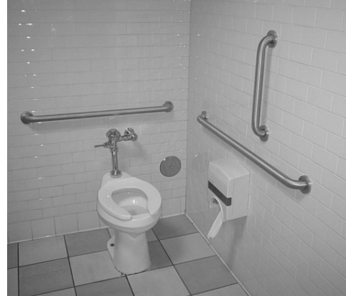
Figure 3-1.7b Grab bar picture; codes vary by location – Minnesota requires a vertical bar as shown above.
