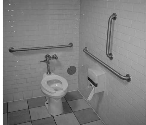
Figure 4-1.7b Grab bar picture; codes vary by location – Minnesota requires a vertical bar as shown above.
