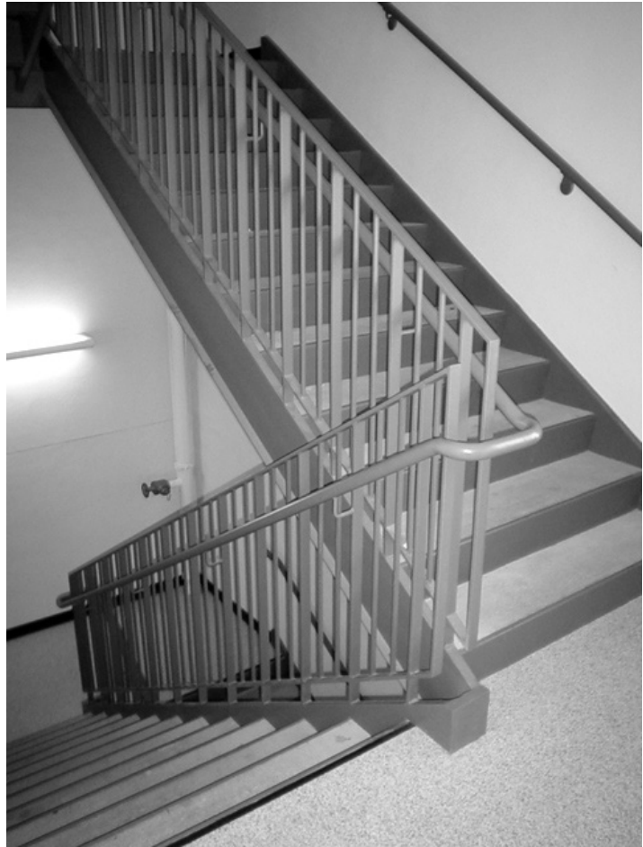
Utilitarian Stair Example Durable, average cost stair with simple design
