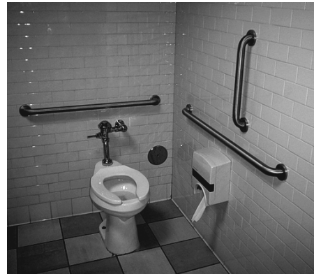
FIGURE 4-1.6B Grab bar picture Codes vary by location; some US states require a vertical bar as shown above.
